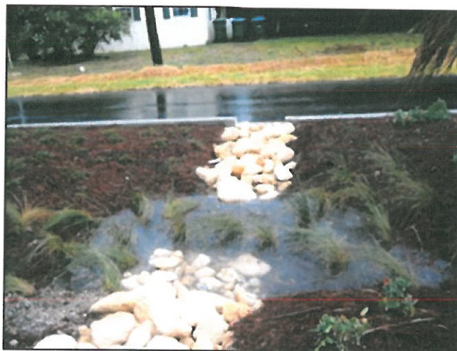
Figure 2. Energy Dissipaters and Sediment Sumps
