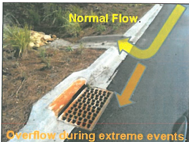
Figure 1. Curb Cuts with High-Flow Bypass
