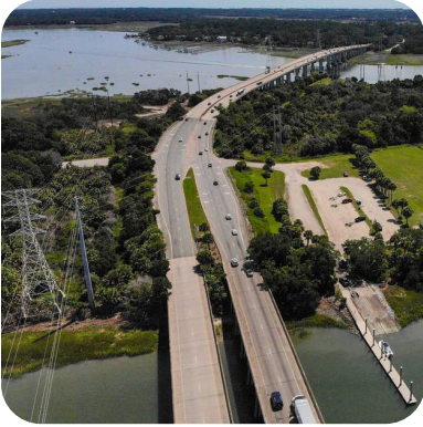
Aerial view of current bridges headed into Hilton Head
