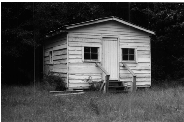
Image 46. The Coffin Point Praise House in 1997. Since this photograph, portions of the building's rough-cut weatherboard were replaced with machine-cut weatherboard. Source: South Carolina Department of Archives and History 1997.
