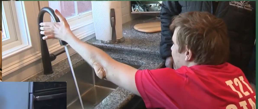
Smart Homes Wheelchair Height Sink and Touch Faucet
