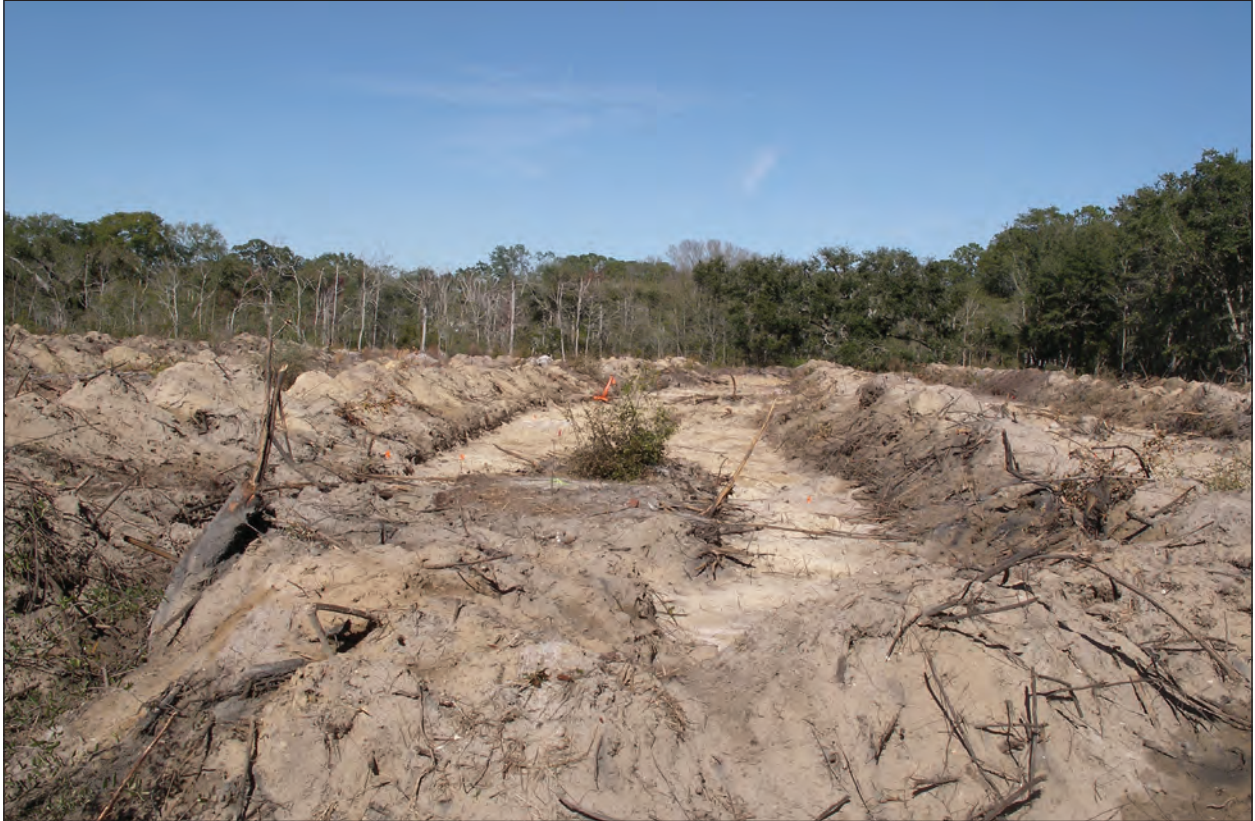
Figure 4.18 Scrape 3 (northeast view).
