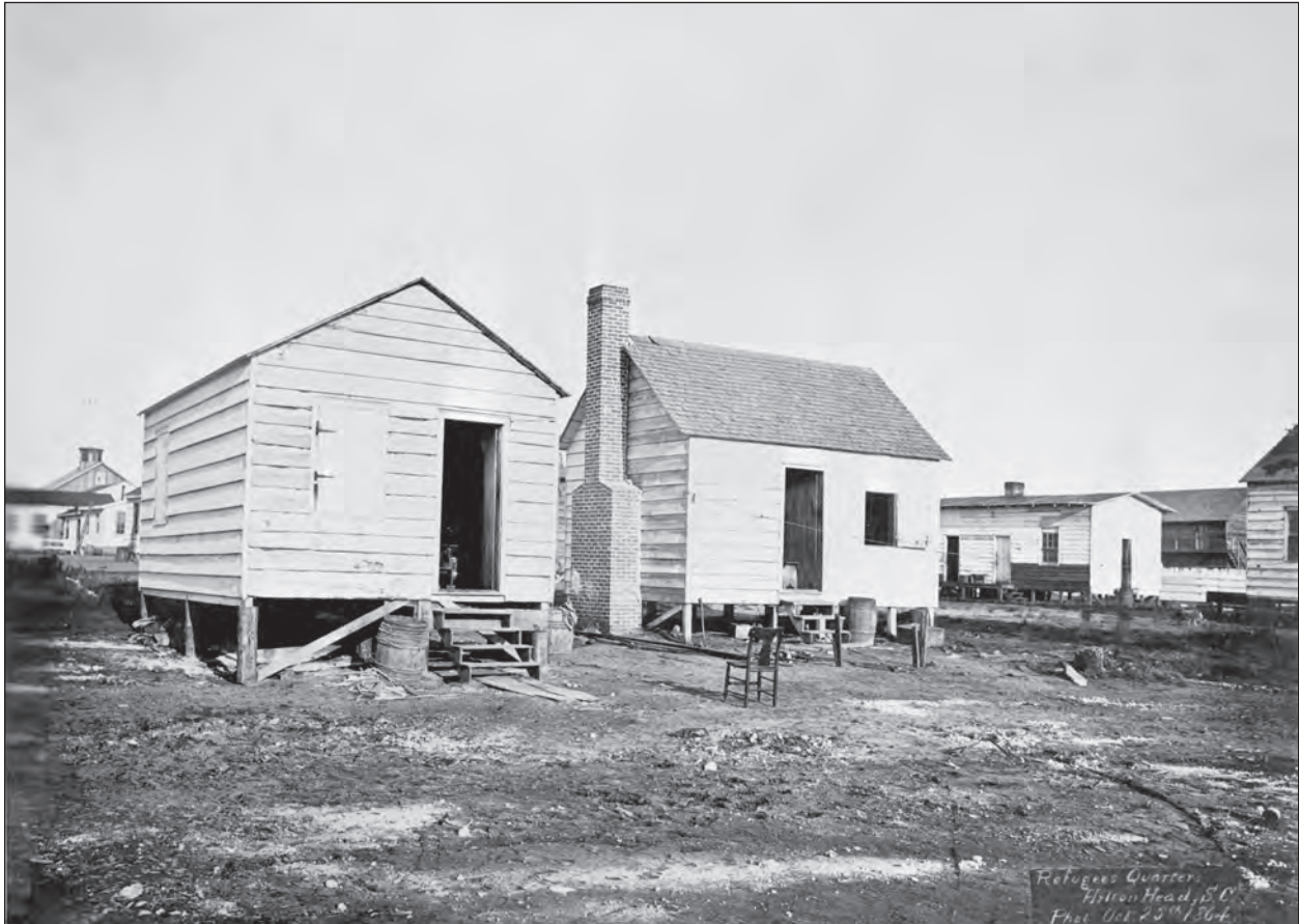
Figure 2.10 Of the few photographs taken of houses at Mitchelville; few houses appeared to have traditional chimneys; many had stove flues (NARA photograph 165-C-137).
