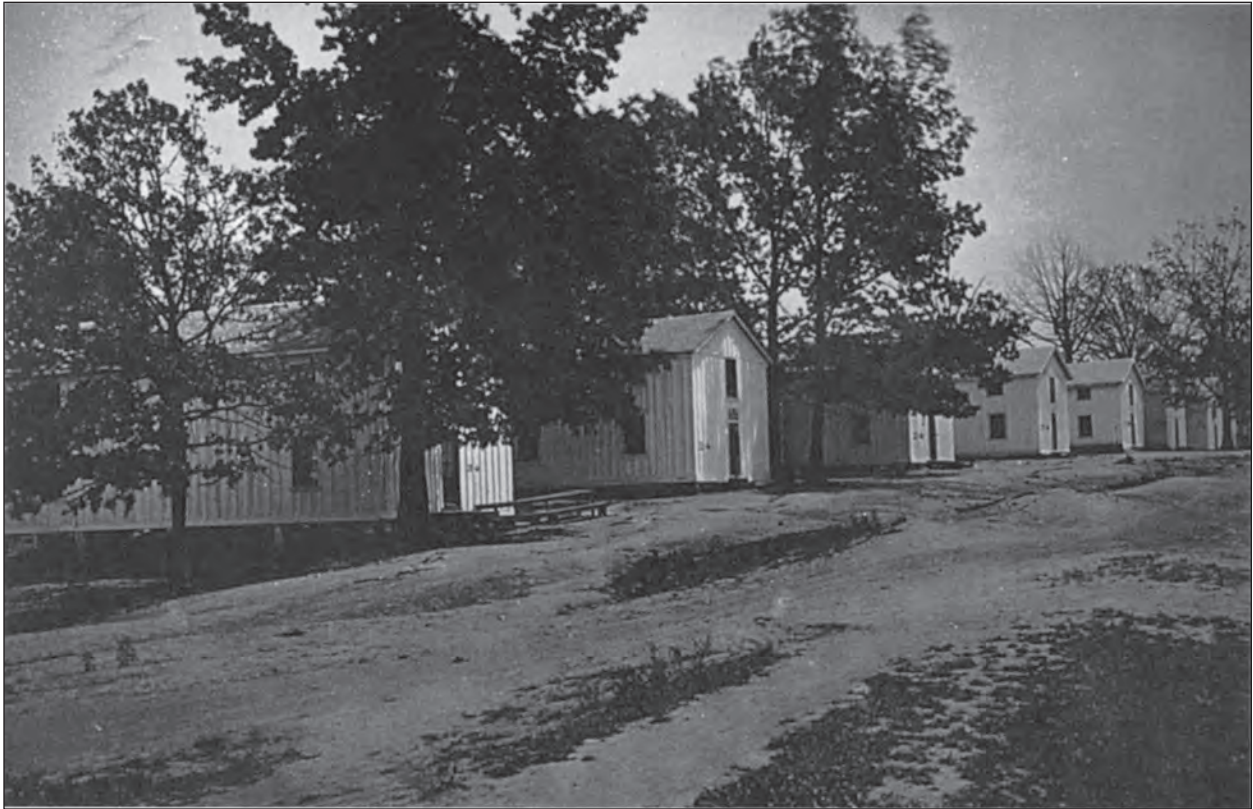
Figure 6.9 A neat row of houses at Mitchelville, showing a more substantial structure at one and one-half stories (McCracken 1993).
