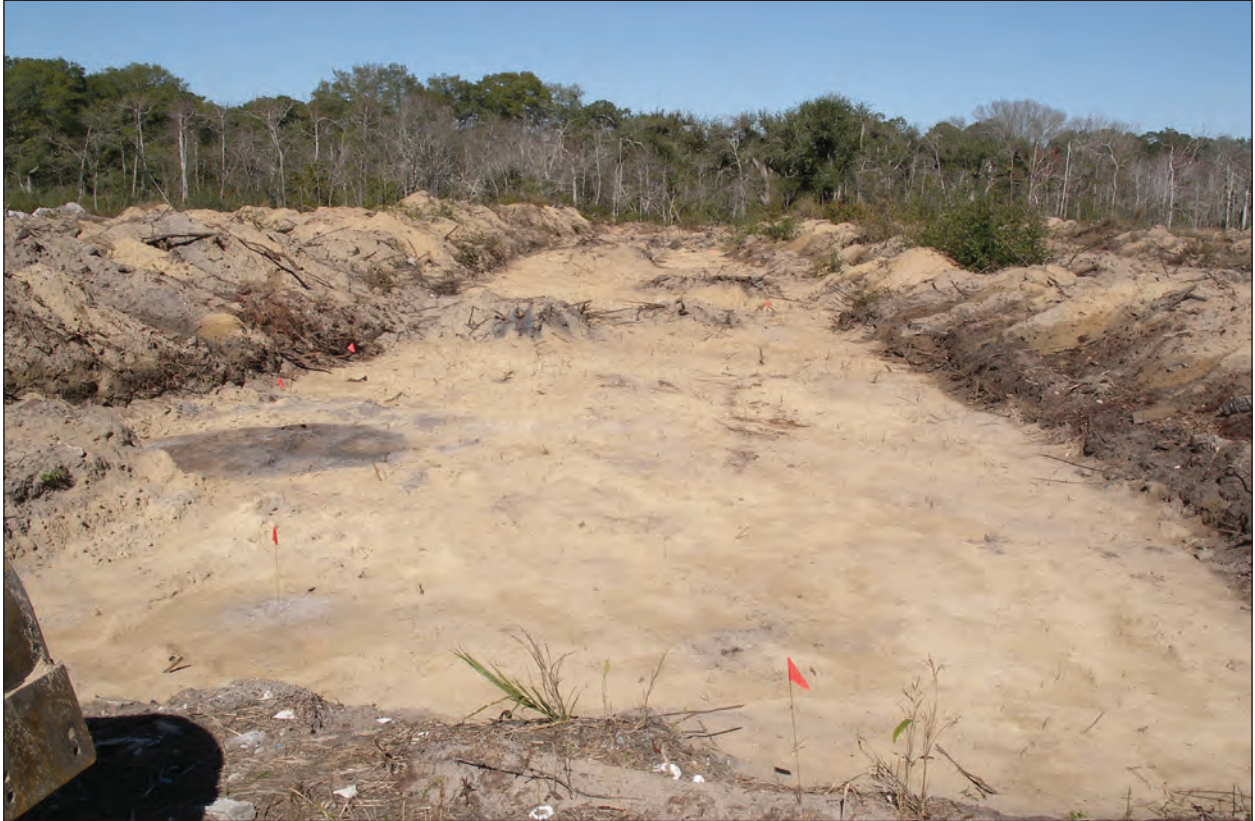
Figure 4.33 Scrape 9, northeast view.
