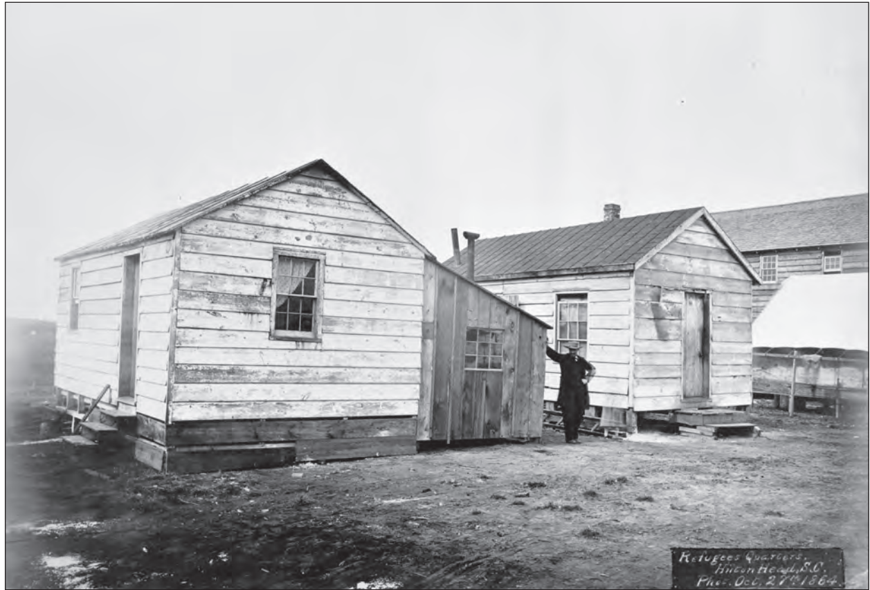
Figure 6.4 Refugee quarters at Hilton Head, October 27, 1864 (NARA photograph 165-C-138).
