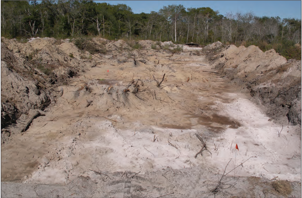
Figure 4.39 Scrape 11, northeast view.
