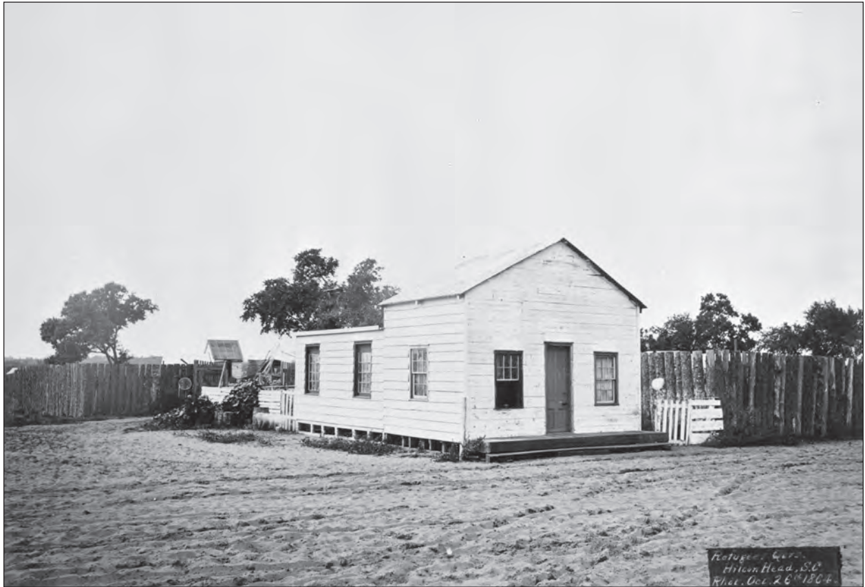
Figure 6.3 Refugee quarters at Hilton Head, October 26, 1864 (NARA photograph 165-C-135).
