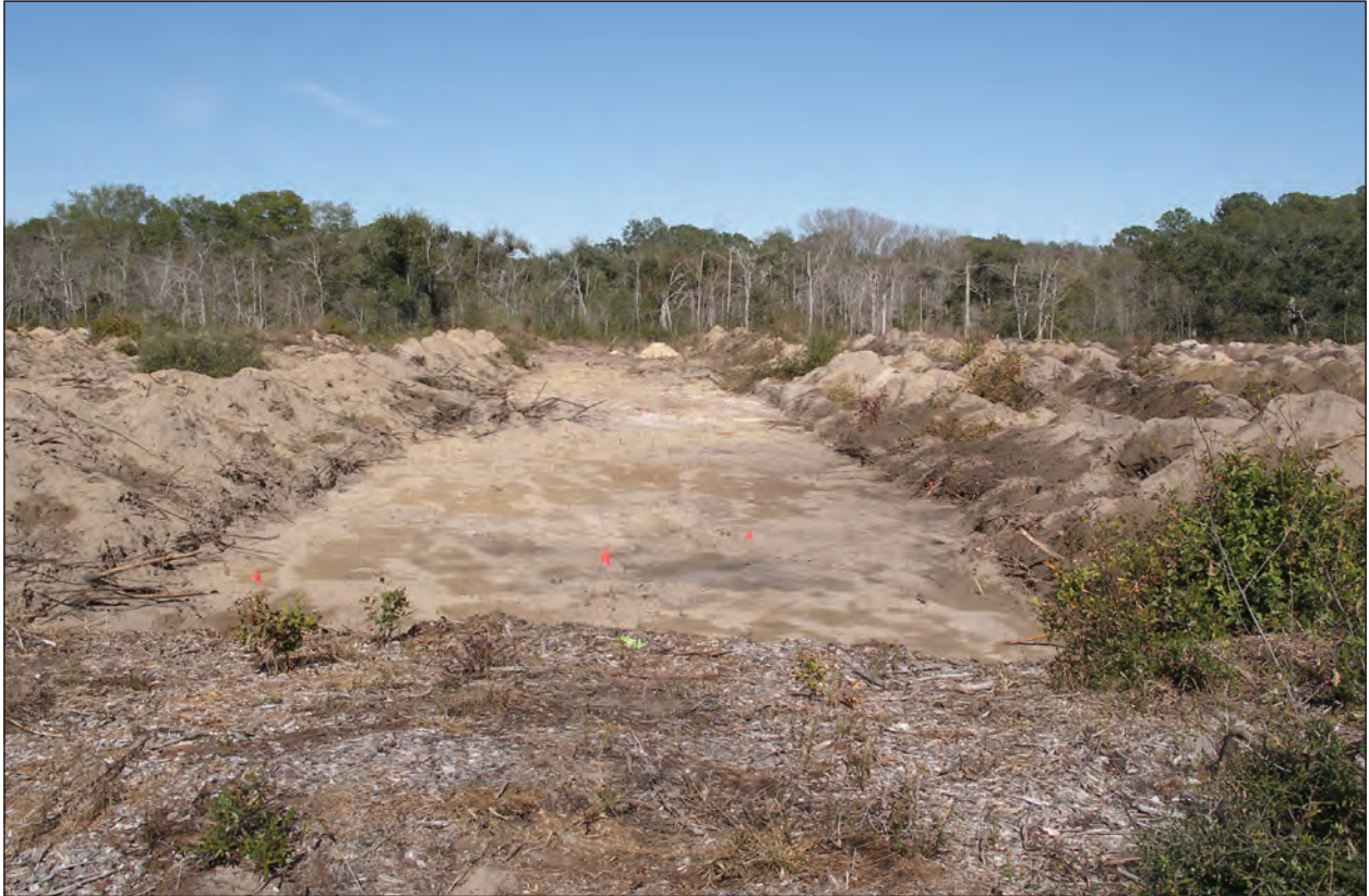
Figure 4.30 Scrape 7 (northeast view).
