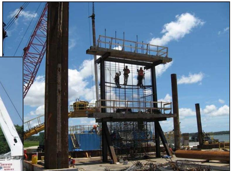
Construction Workers Tying Rebar for Bridge Construction
