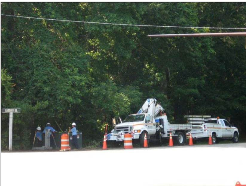
Palmetto Electric Working on Transformers at Gardner Drive
