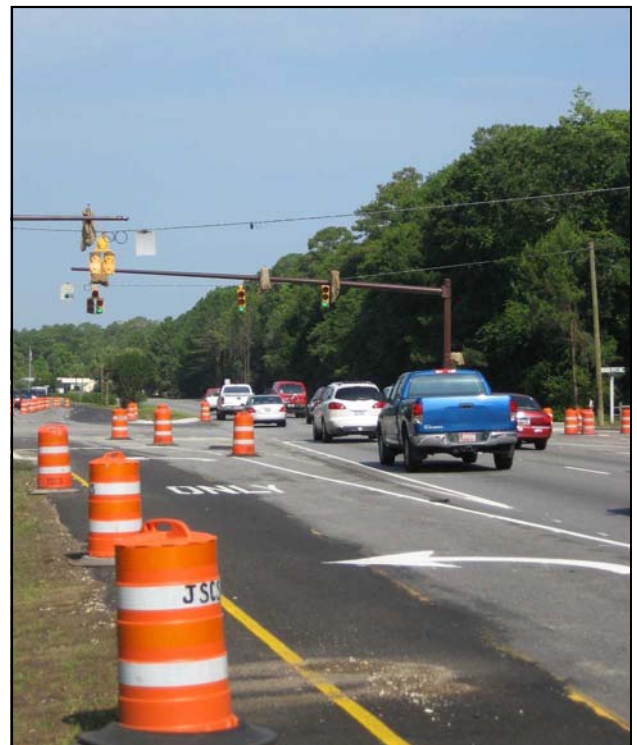
Widened Turn Lane from William Hilton Parkway to Beach City Road
