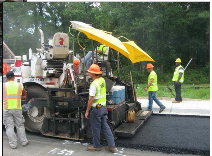
Installing Base Course
