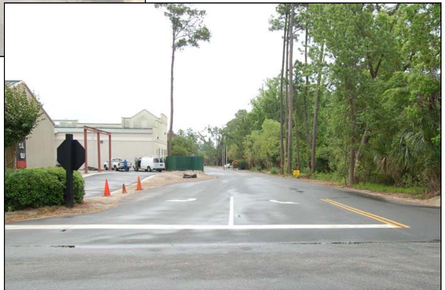
Completed Paving for New Frontage Road
