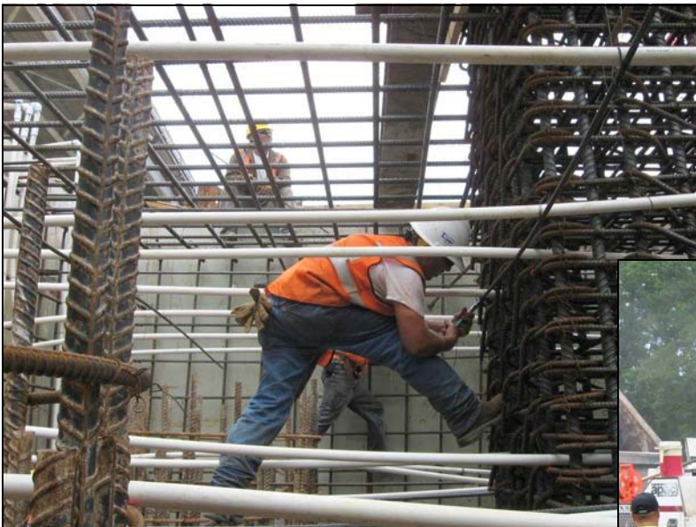
Bridge Crew Tying Rebar for the Bridge
