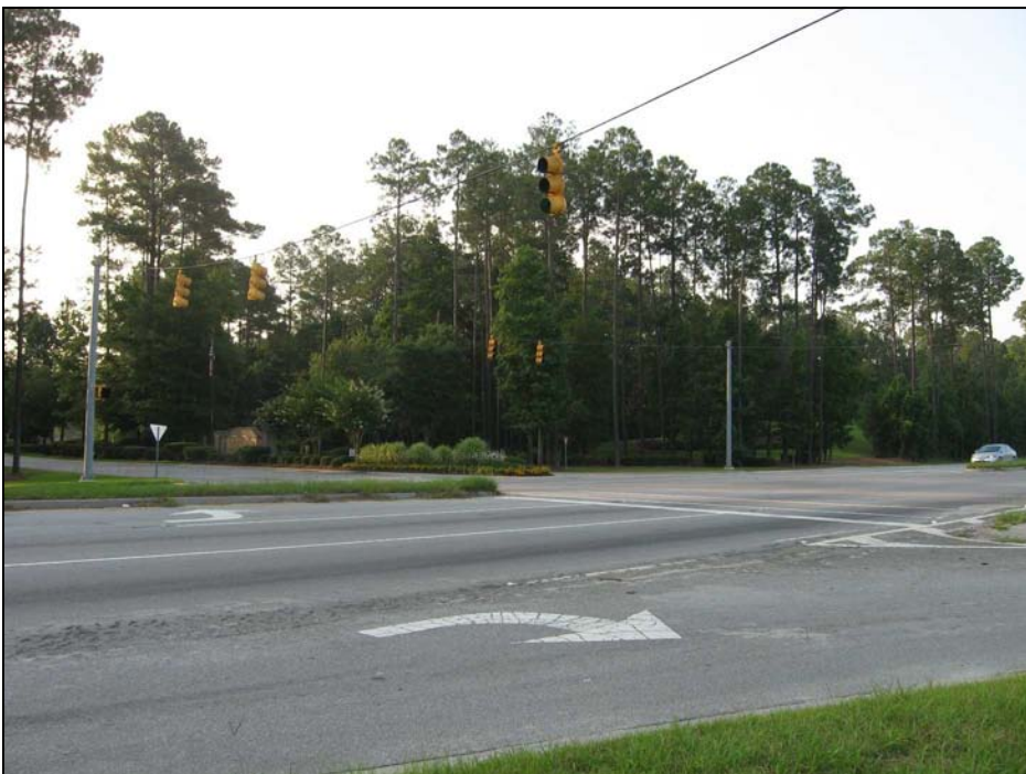
Alligator Cracking at the Intersection of Tide Watch Drive and SC 170
