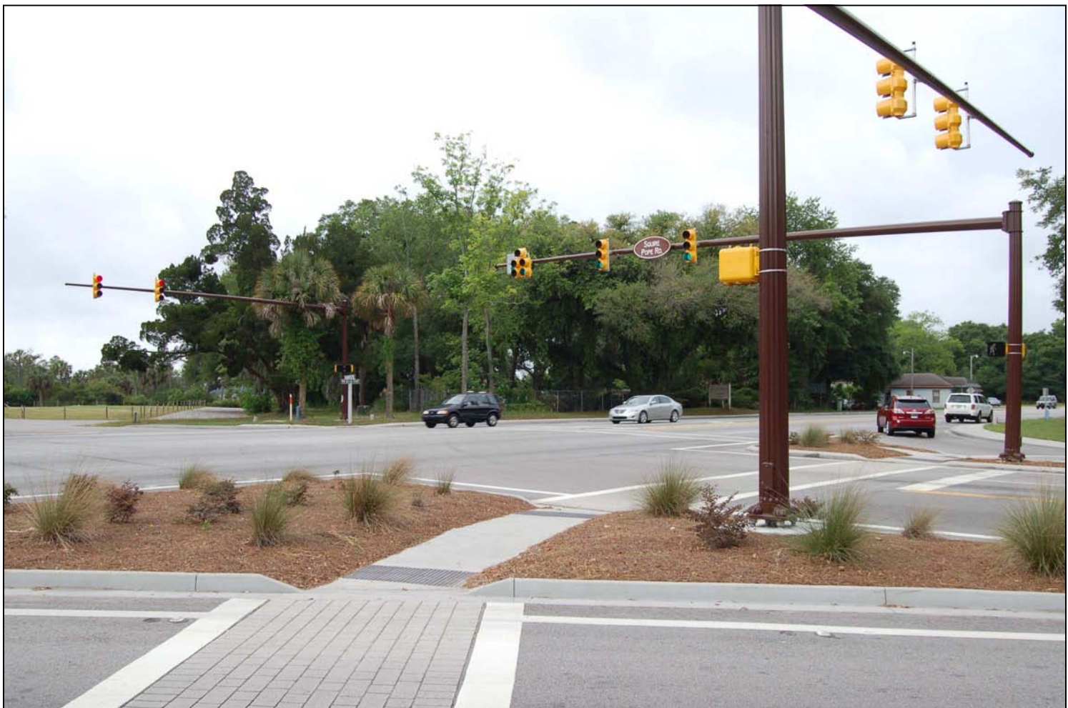
Realignment of the Intersection of US 278 and Squire Pope Road with New Mast Arm Traffic Signals
