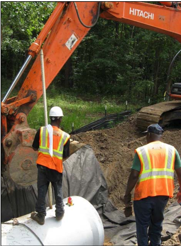
Installation of 36 Inch Storm Drain
