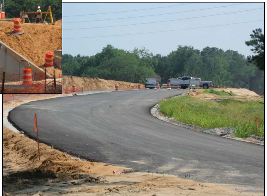
Ramp at the Gardens Corner Intersection
