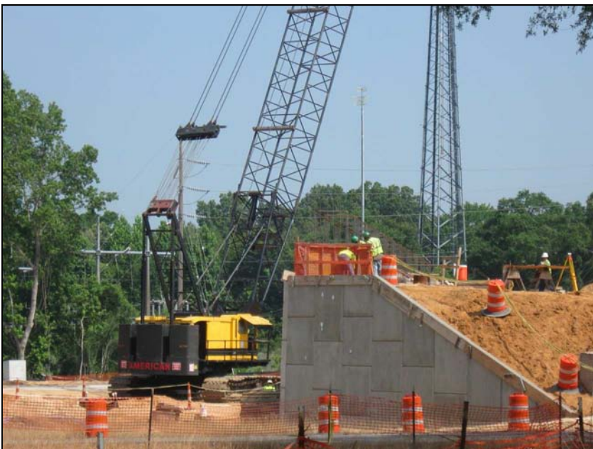
Construction at the Gardens Corner Intersection
