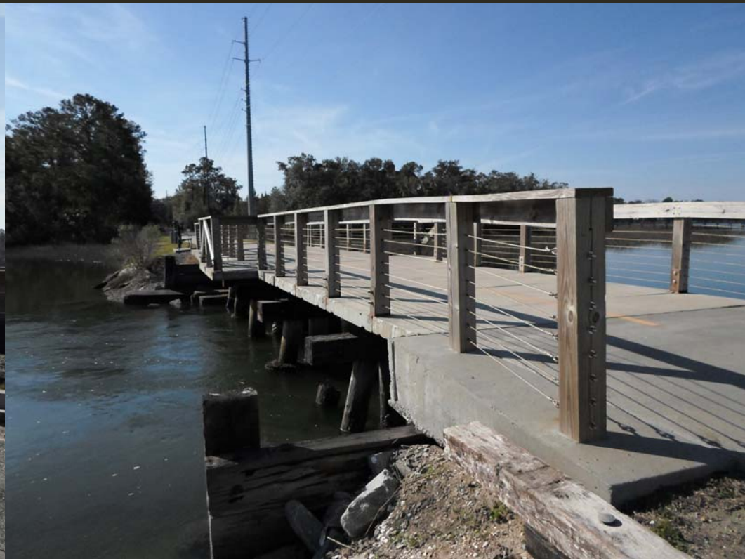
Spanish Moss Trail Boardwalk – Side View
