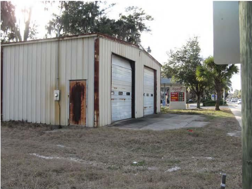
METAL BUILDING LOOKING WEST
