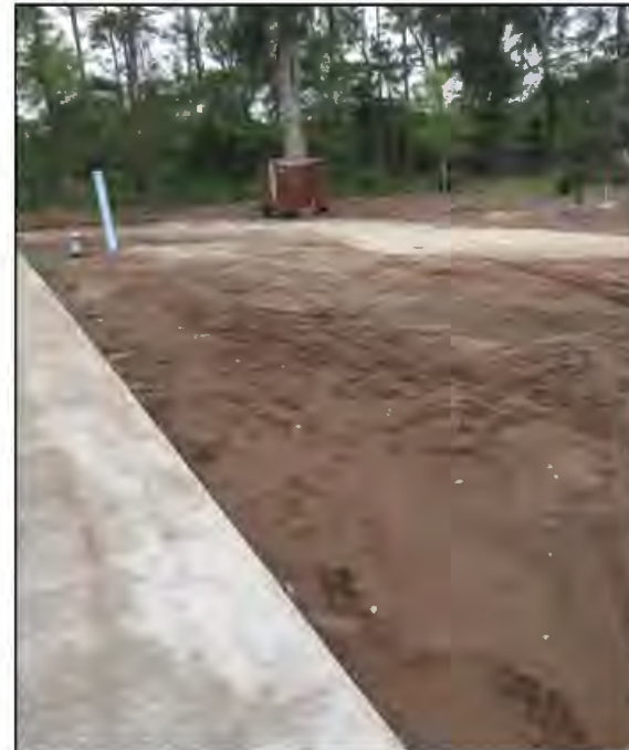
Erosion and elevation and change
