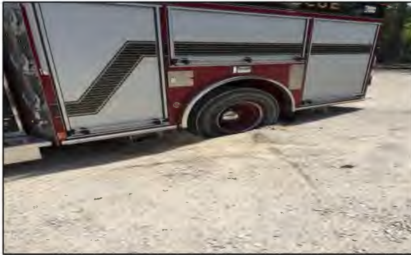
Surface degraded and vehicle stuck
