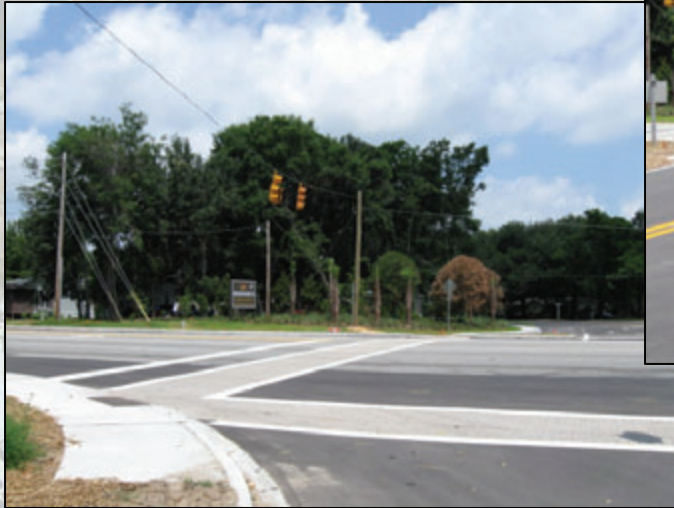
Crosswalk for Pedestrian Access Across Highway 278
