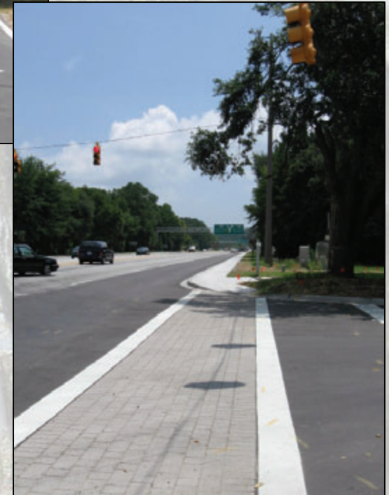
Sidewalk and Crosswalks Complete
