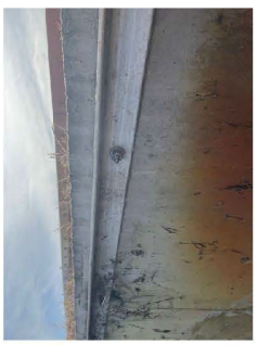
All "A" grate structures, A3, Midfield and A5 on Alpha Taxiway side have 2"x2" aluminum angle supported with bolts on the structure.
